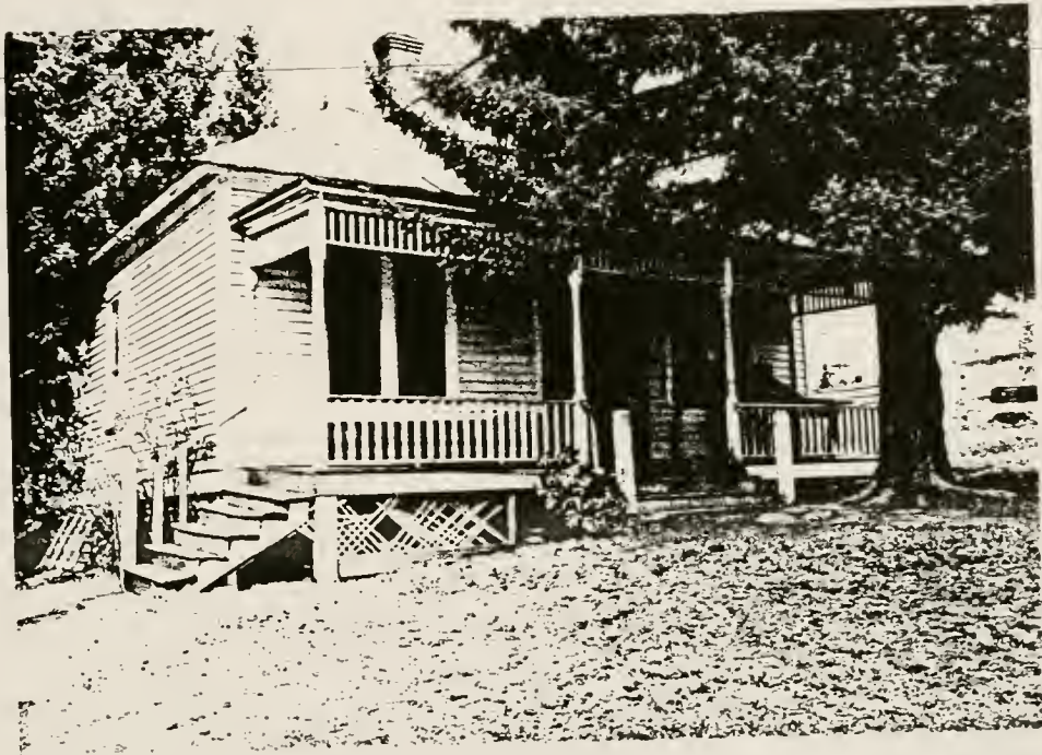
Figure 189. Harry Bush guesthouse (structure #67), northeast view.
